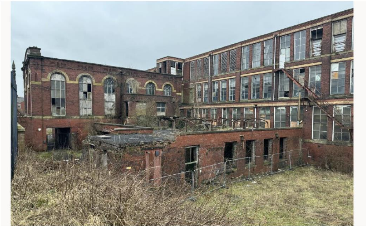
Figure 12 – Photograph of Boiler House adjoining the Engine House and main Mill behind
