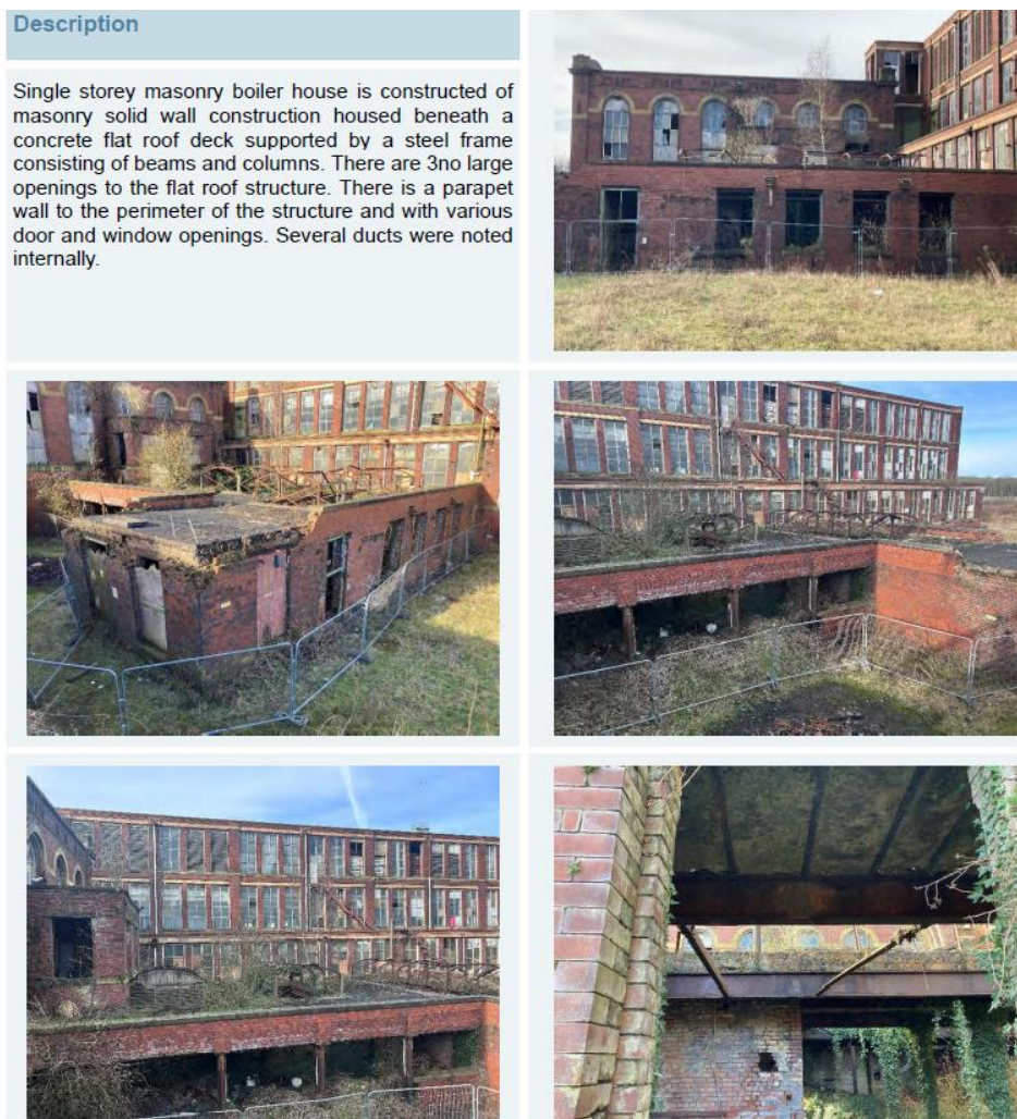
Figure Three – description and site photographs:
