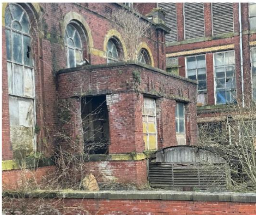
Figure 18 – Photograph of Engine Room Extension
